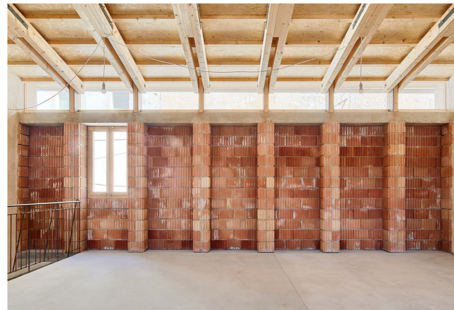
MUNICIPAL BUILDING (AULETS ARCHITECTES)
