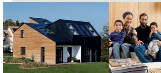
Maison Air et Lumière, France 2011 Daylight and natural ventilation create energy efficiency and great indoor comfort – particularly during hot summer months.
